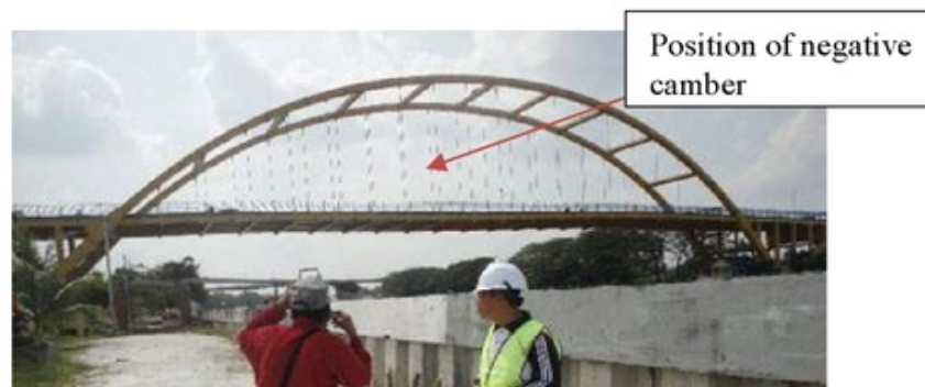
Fig. 3 Measuring camber position bridges with total station
